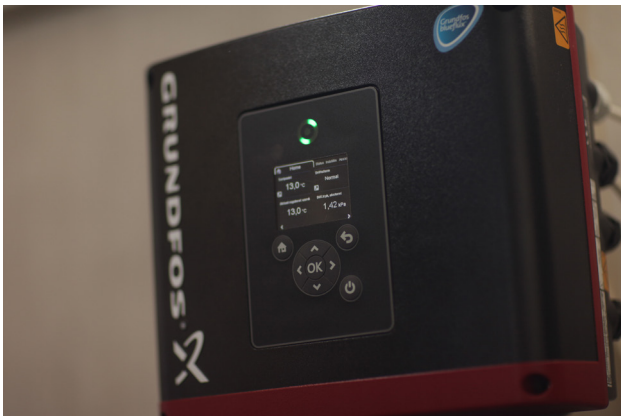
A close up of the TPE3 pump installed at Langenæs.
