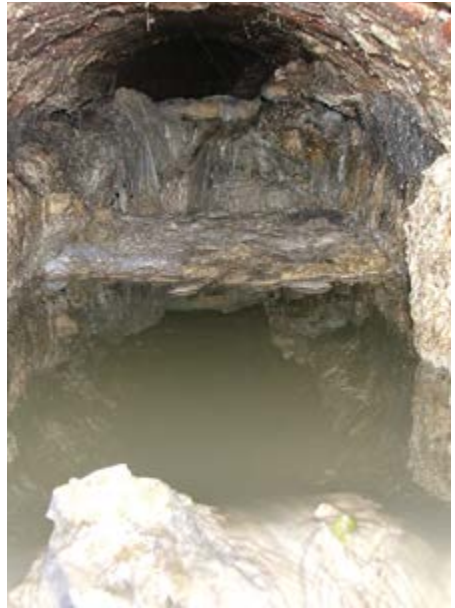
Example of fat, grease and debris build-up in a large sewage pipe.
