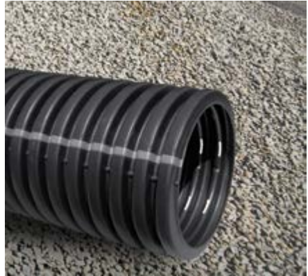
Drain pipe embedded in a gravel trench.
