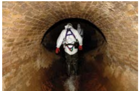
Wastewater inspection in a large sewage main pipe.
